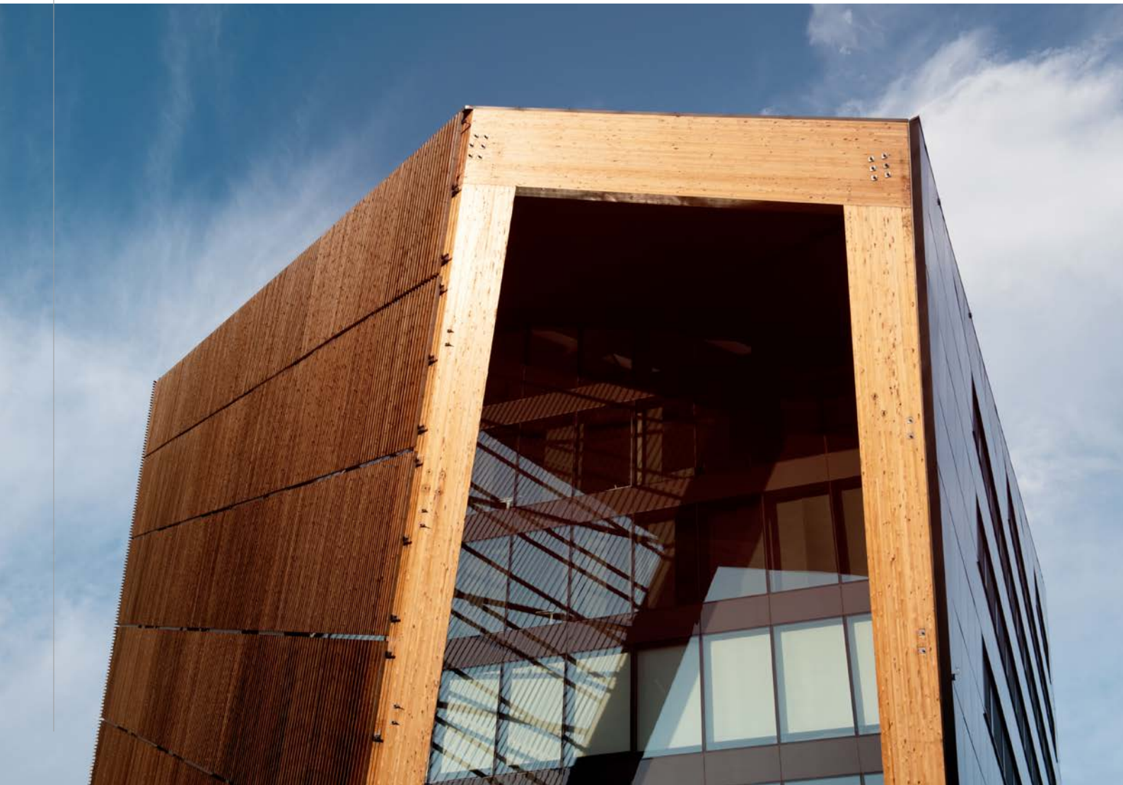
Benchmark by Thermory thermo-pine cladding Powerhouse Telemark in Norway Designed by Snøhetta Architects. Photo by Jeanett Teigen, BLAAtime
